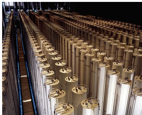
Figure 3. Picture of centrifuge plant in practice.
