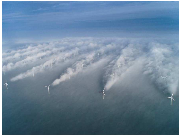
Figure 13. Fog formation in the wake of wind turbines at sea.
